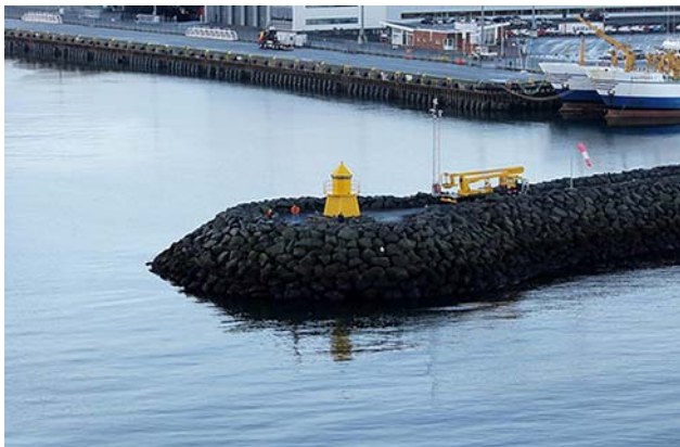
Skarfagarðs Light at Reykjavik Breakwater
