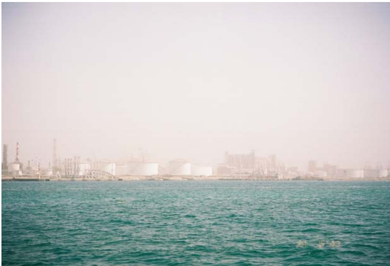
Mina Jabal Ali—Tanker Berth No. 3 (left) and Tanker Berth No. 1 (right)
