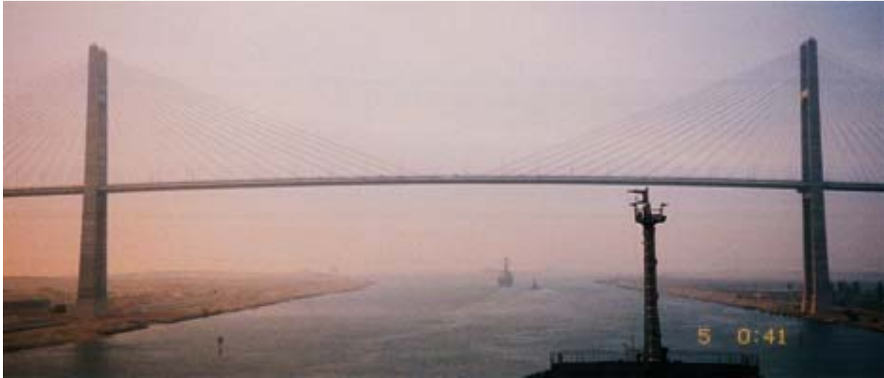
The International Peace Bridge (Al Qantarah Bridge) from N
