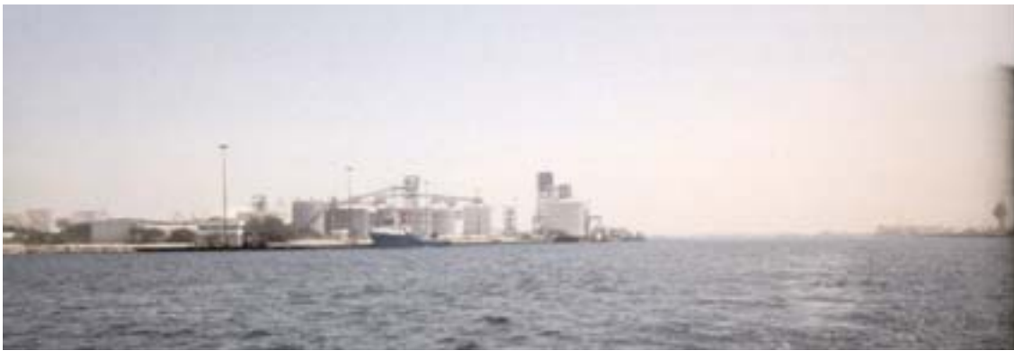
Mina Jabal Ali—Tanks and silos at the entrance to the Outer Basin
