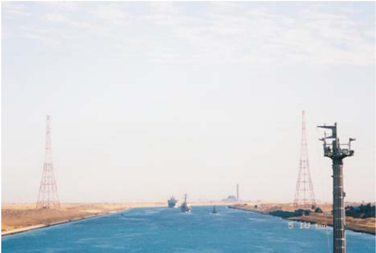
Power lines near Km 153.0 from N
