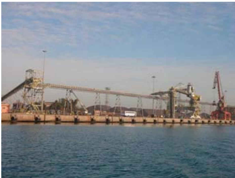
Courtesy of Qatar Petroleum Mesaieed Port Development Mesaieed—QASCO Berth No. 3
