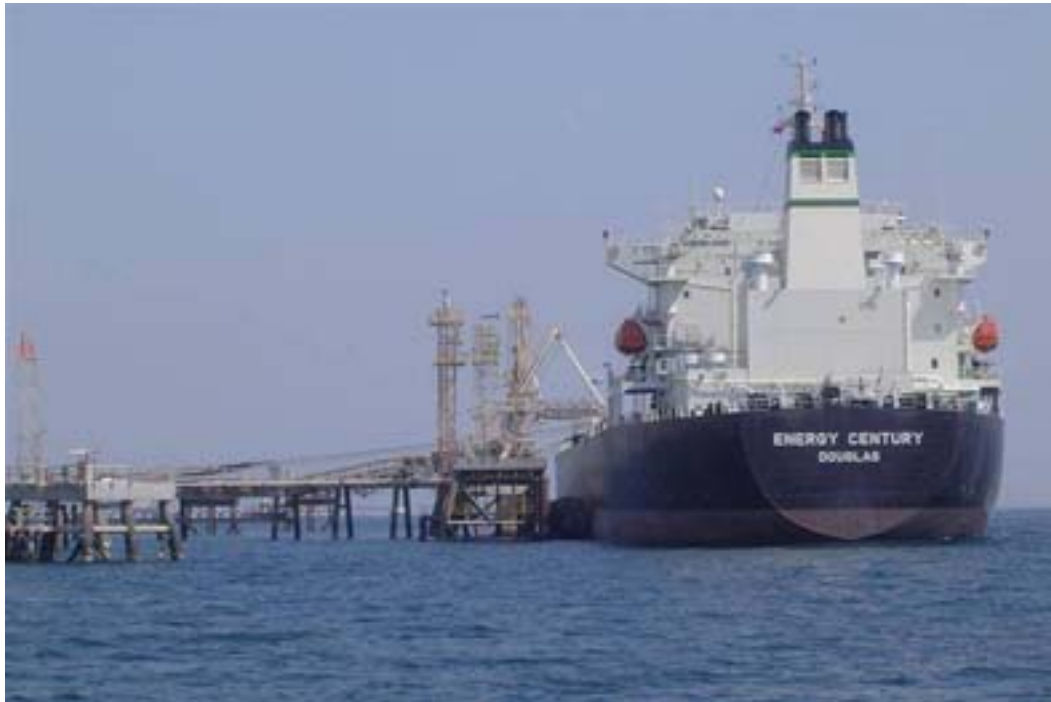
Courtesy of Qatar Petroleum Mesaieed Port Development Mesaieed—NGL Jetty
