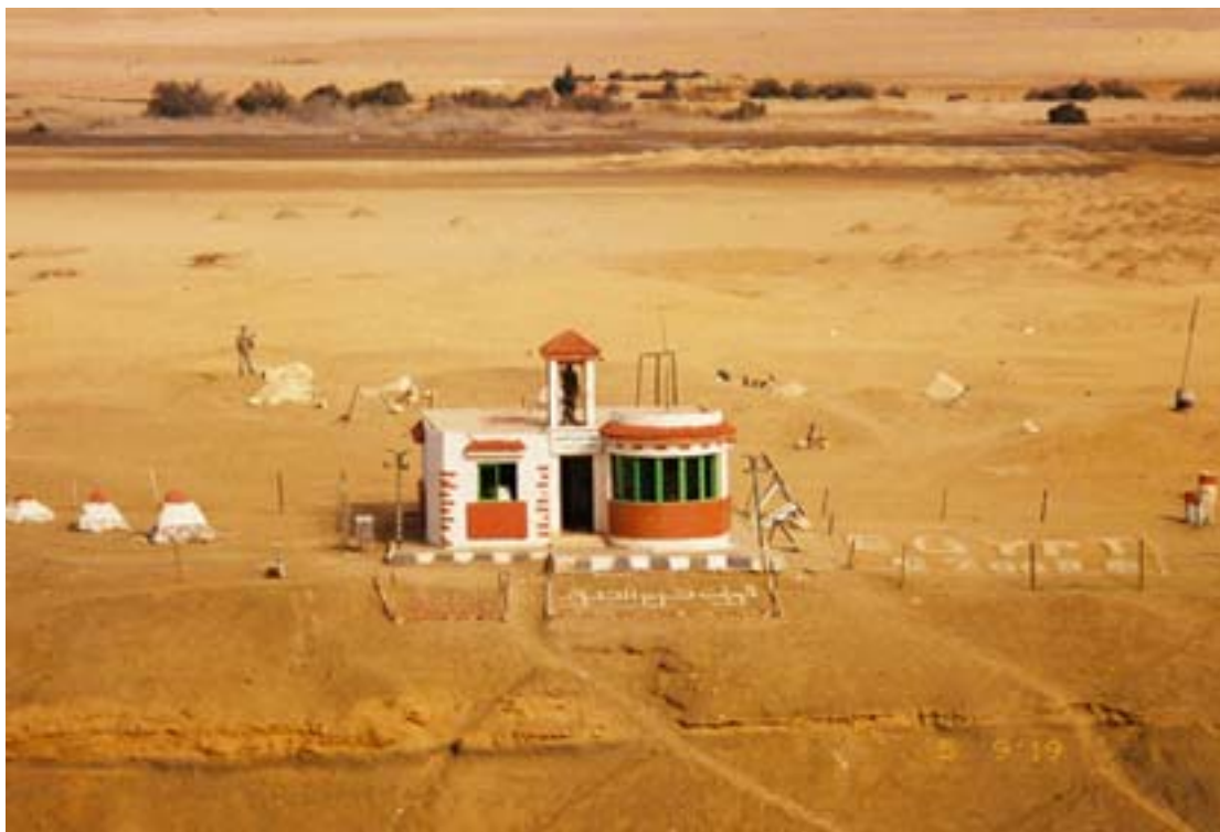
Suez Canal—Typical Security Facility
