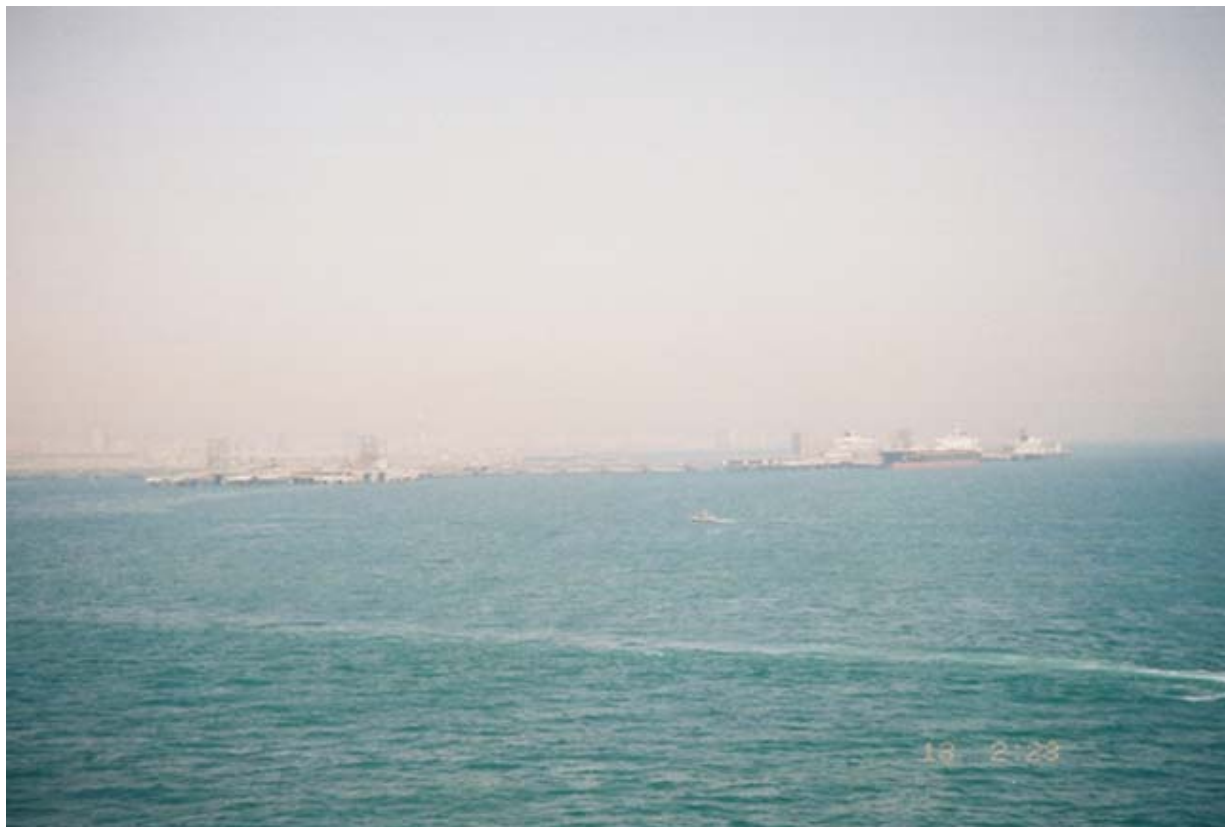
Mina al Ahmadi—New Oil Pier from SE
