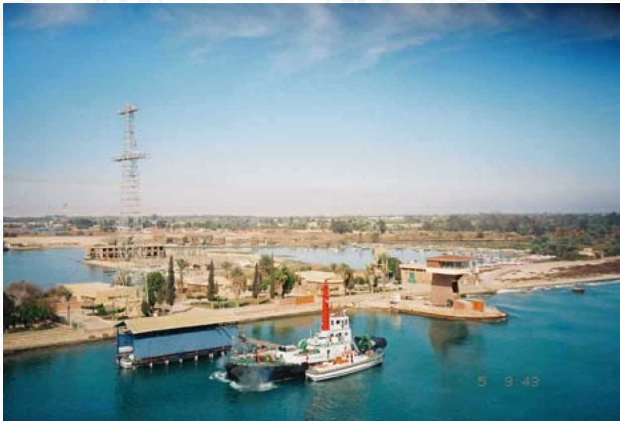
Suez Canal—Typical Signal Station
