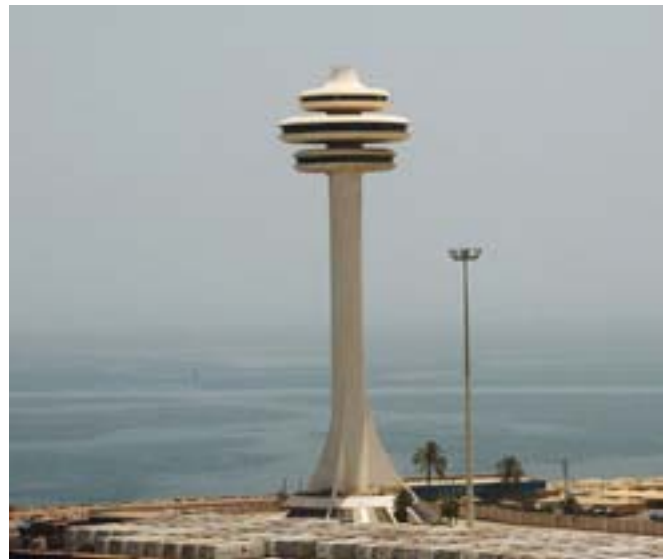
Dammam Control Tower
