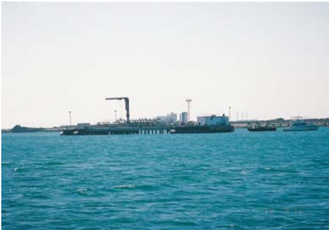
Aden Inner Harbor—Bunker pier close W of Aden Container Terminal
