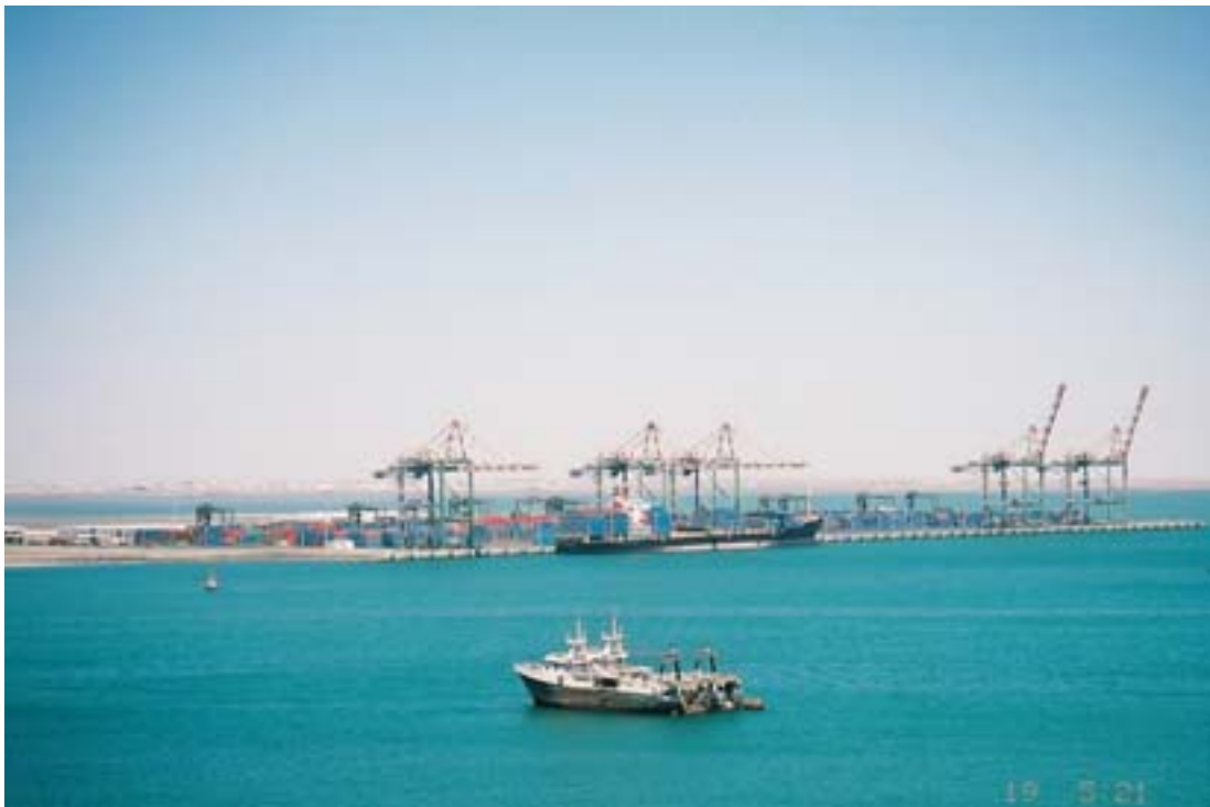
Aden Inner Harbor—Aden Container Terminal
