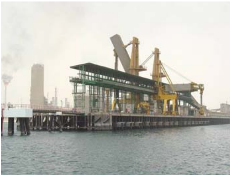
Courtesy of Qatar Petroleum Mesaieed Port Development Mesaieed—QAFCO Berth No. 1 (charted as Berth No. 20)
