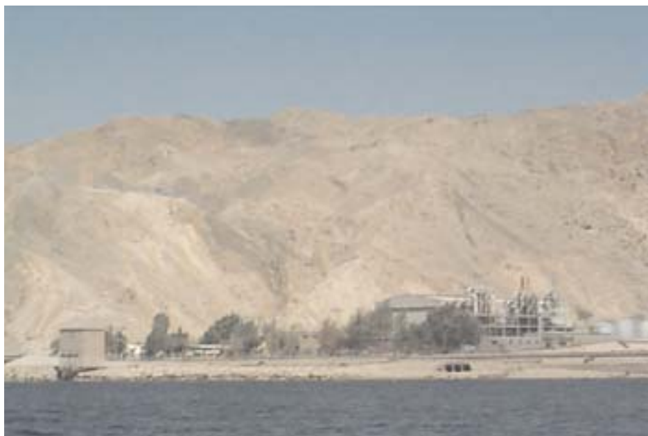
Al Aqabah—Power Station
