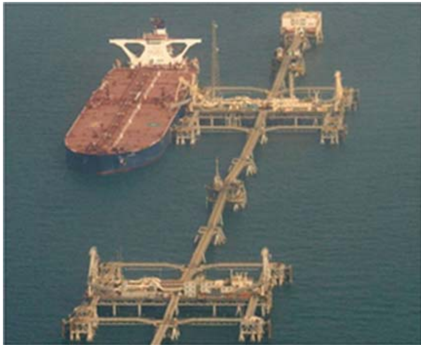
Al Basra Oil Terminal
