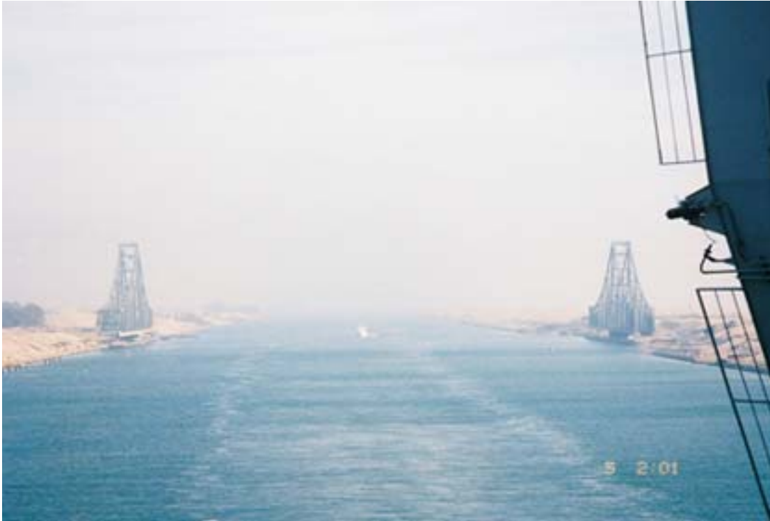
El Firdan Bridge from N
