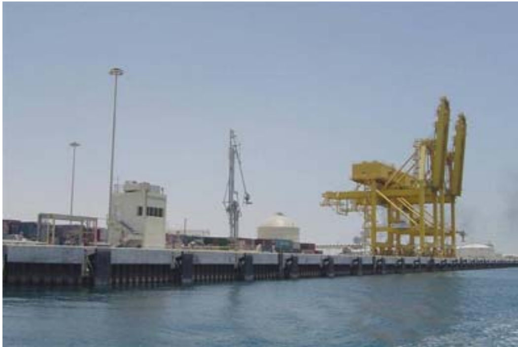
Courtesy of Qatar Petroleum Mesaieed Port Development Mesaieed—Q-CHEM Berth No. 1 and Q-CHEM Berth No. 2
