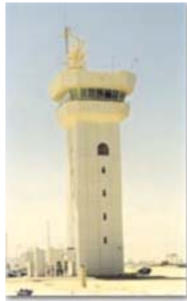
Ras Laffan—Control Tower
