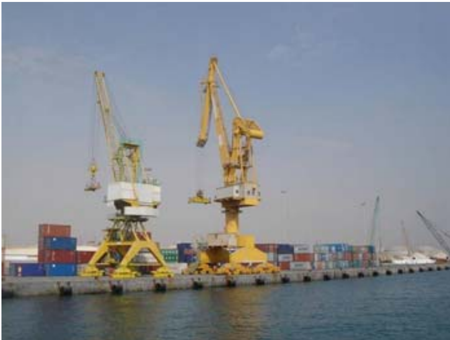
Courtesy of Qatar Petroleum Mesaieed Port Development Mesaieed—QAPCO Berth No. 18
