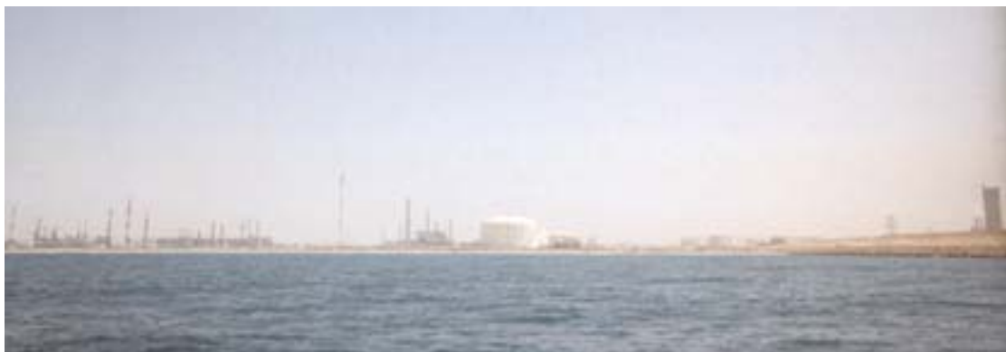
Mina Jabal Ali—Gas Refinery (located E of harbor entrance)
