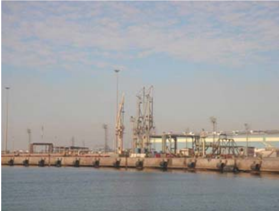
Courtesy of Qatar Petroleum Mesaieed Port Development Mesaieed—QATAX/SEEF Berth No. 4
