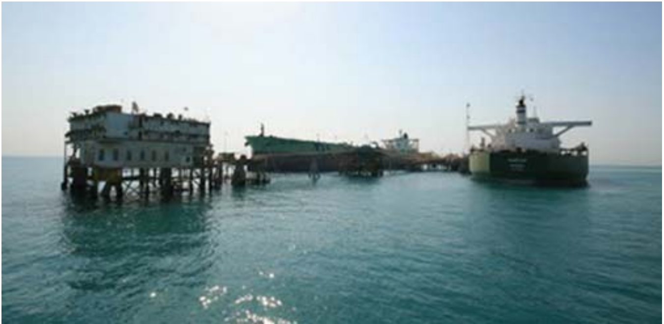
Al Basra Oil Terminal
