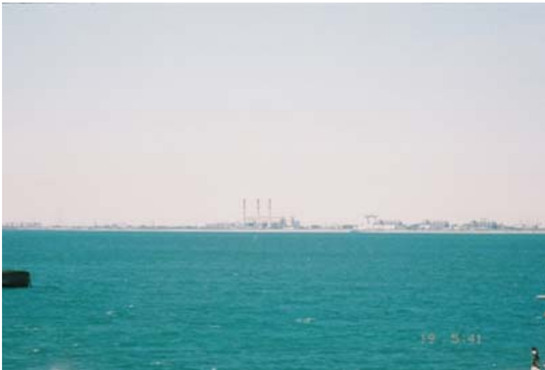
Aden Outer Harbor—Power plant chimney
