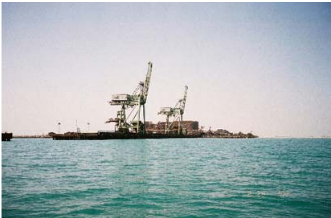
Mina Salman—Bahrain Steel Terminal
