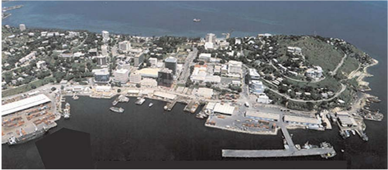
Port Moresby—Main Wharf facing SE
