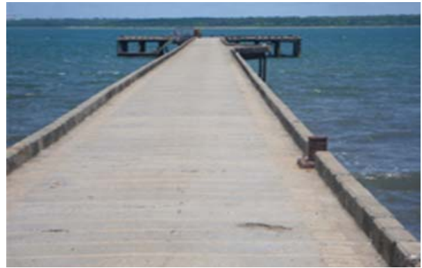
Port of Daru Pier
