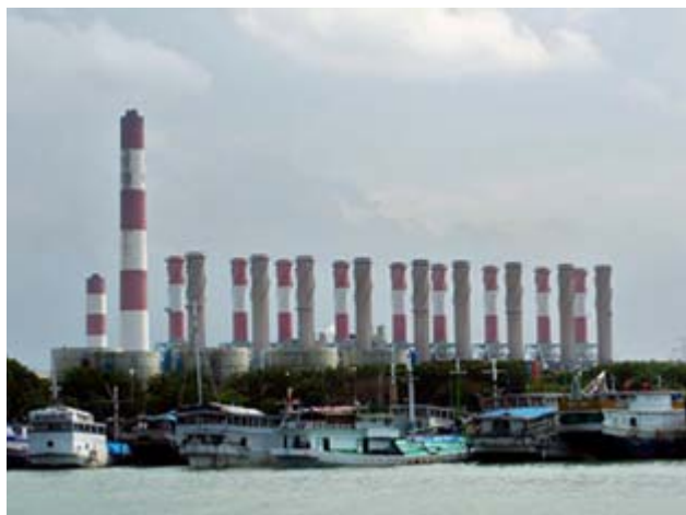
Gresik Power Plant
