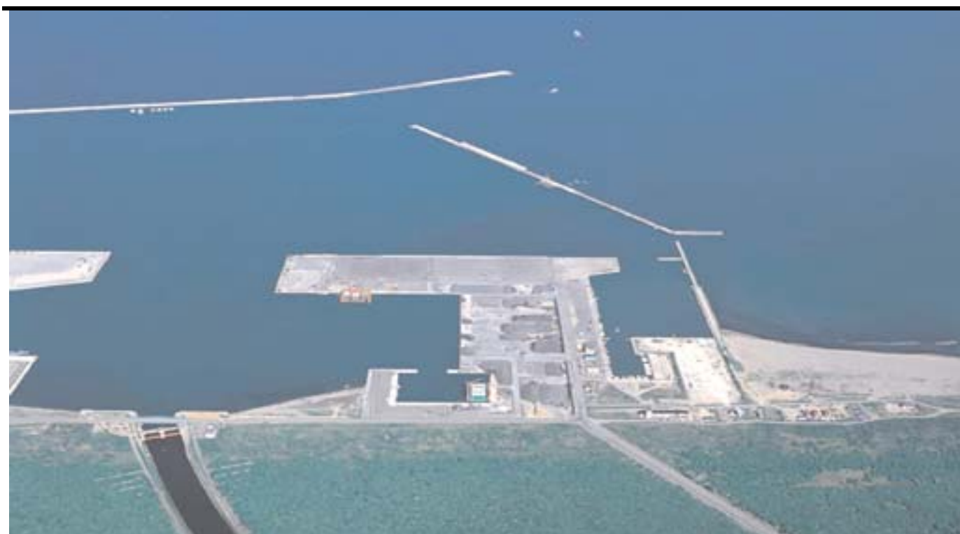
Ishikari Bay New Port—East Wharf
