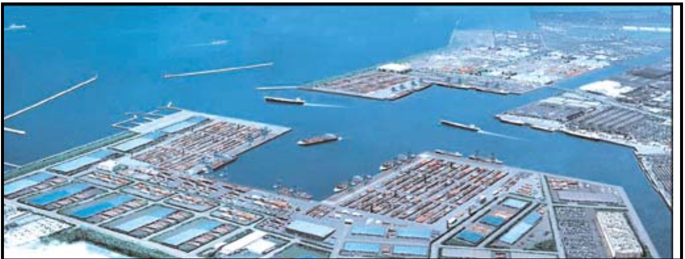
Kitakyushu—Hibiki Port—Hibiki Container Terminal (Future)
