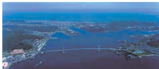
The Hakucho Bridge
