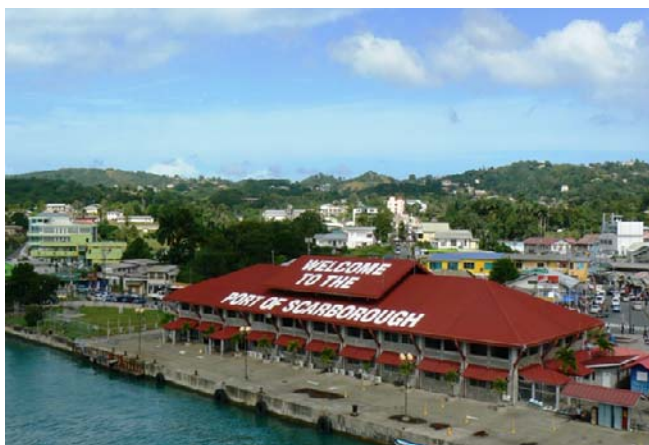
Scarborough Port Terminal
