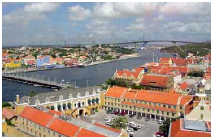
Queen Juliana Bridge (background)
