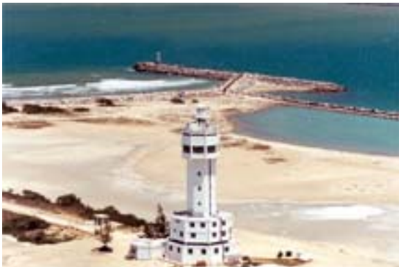
Altamira Light (foreground) and breakwater
