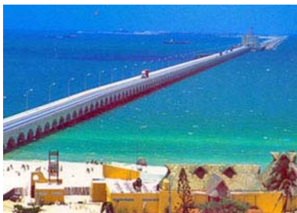
Progreso—Terminal Remota Pier
