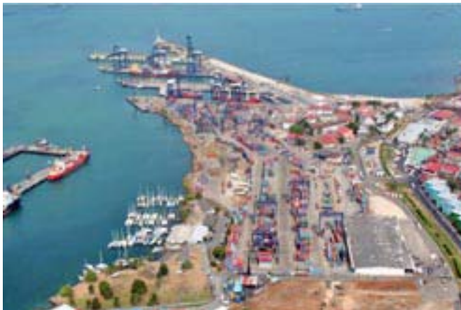
Puerto Cristobal—Piers 6 through 10 (upper) and Pier 16 (left)
