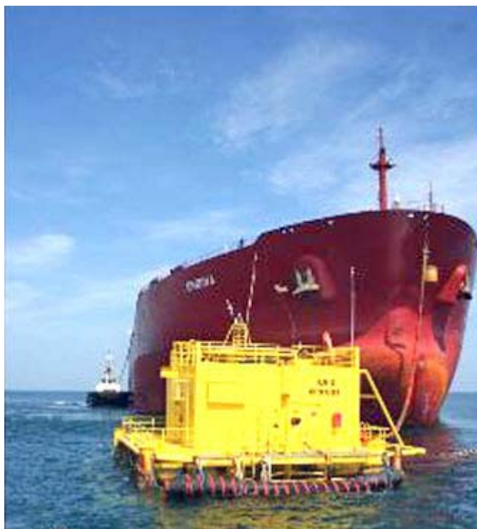
Covenas Tanker Loading Unit (TLU-2)
