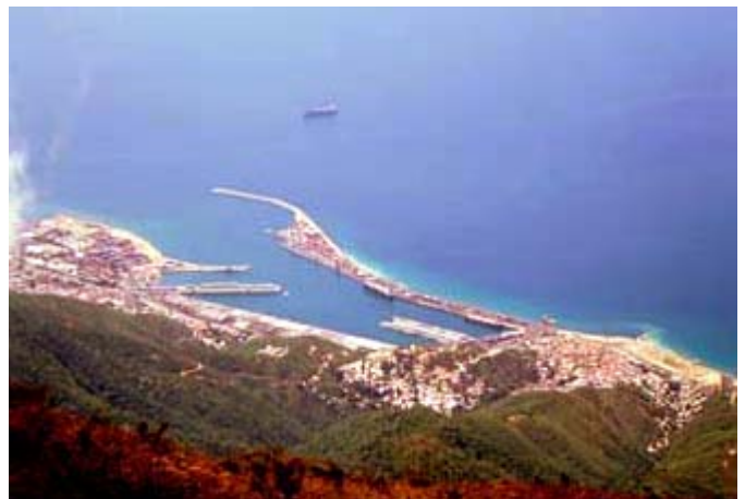
Puerto La Guaira (aerial view)
