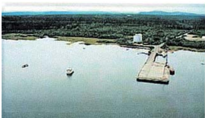
Terrington Basin—Goose Bay (W Dock)
