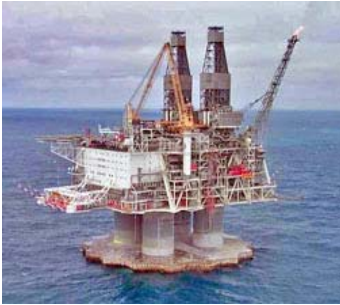
Hibernia Gravity Based Structure
