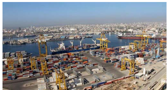
Dakar Port—Container Terminal from NE
