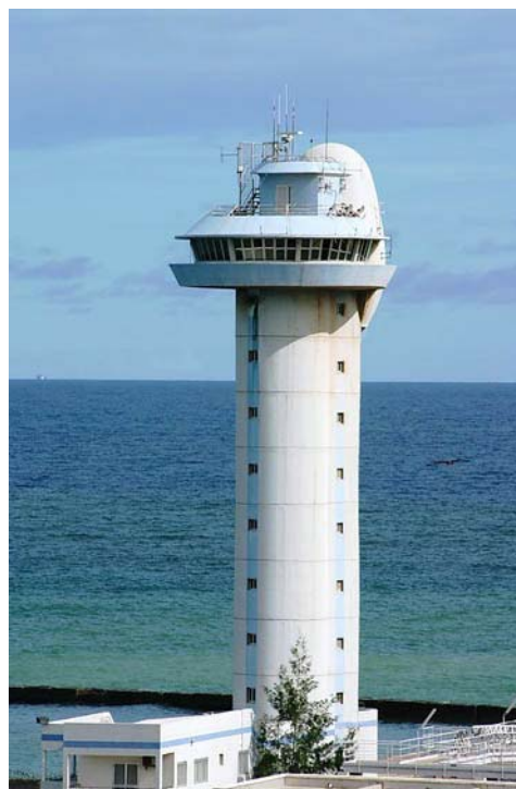
Dakar Harbor Control Tower
