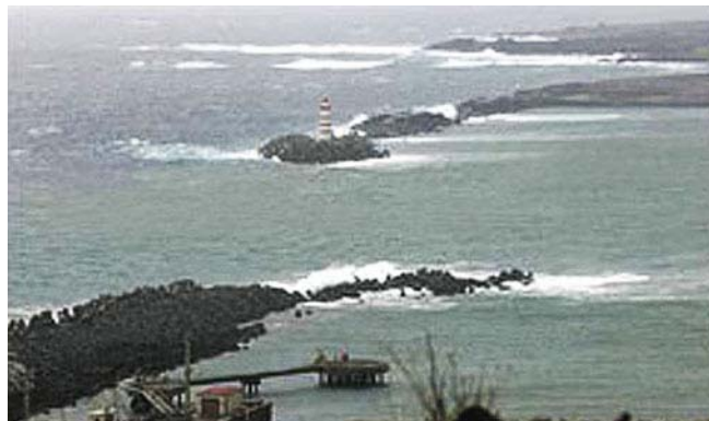
Terceira Light and breakwater
