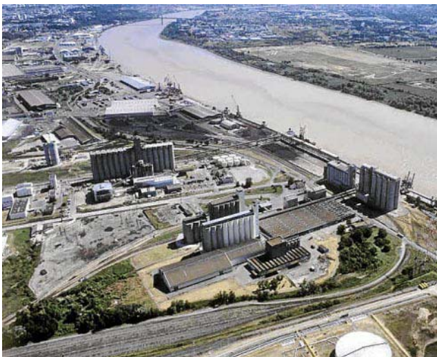
Bordeaux—Dry Bulk and Timber Quay
