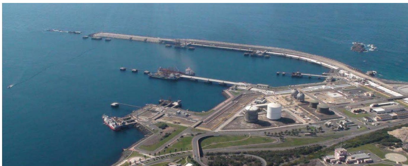
Sines—Oil and Petrochemical Terminal
