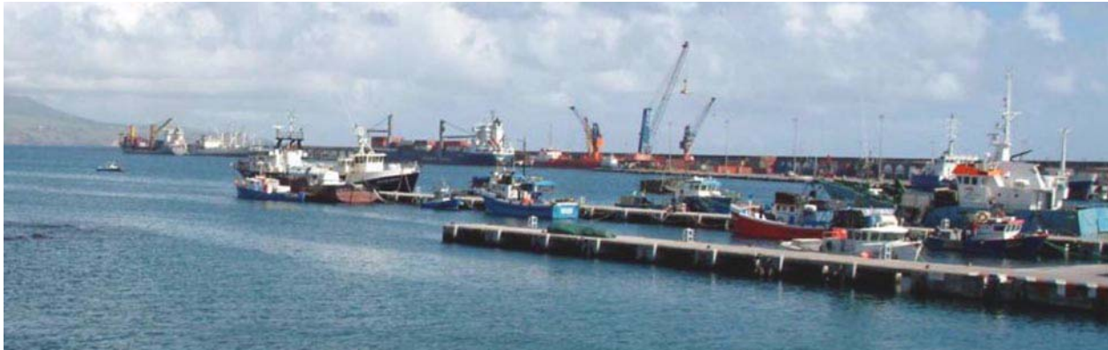
Porto de Ponta Delgada—Commercial Berths
