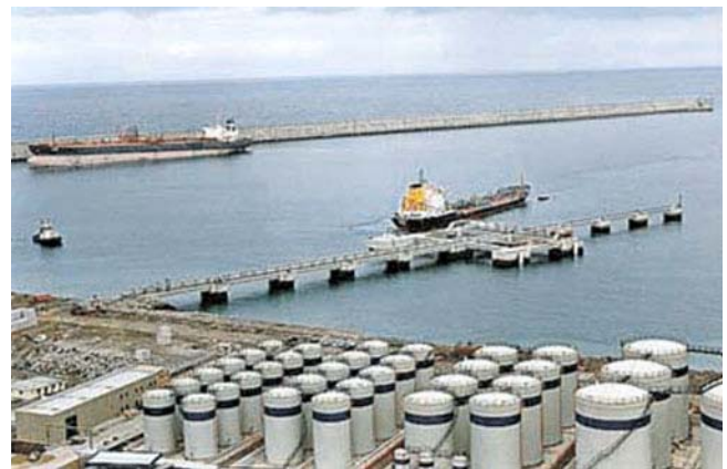
Bilbao—Punta Lucera Breakwater from SE
