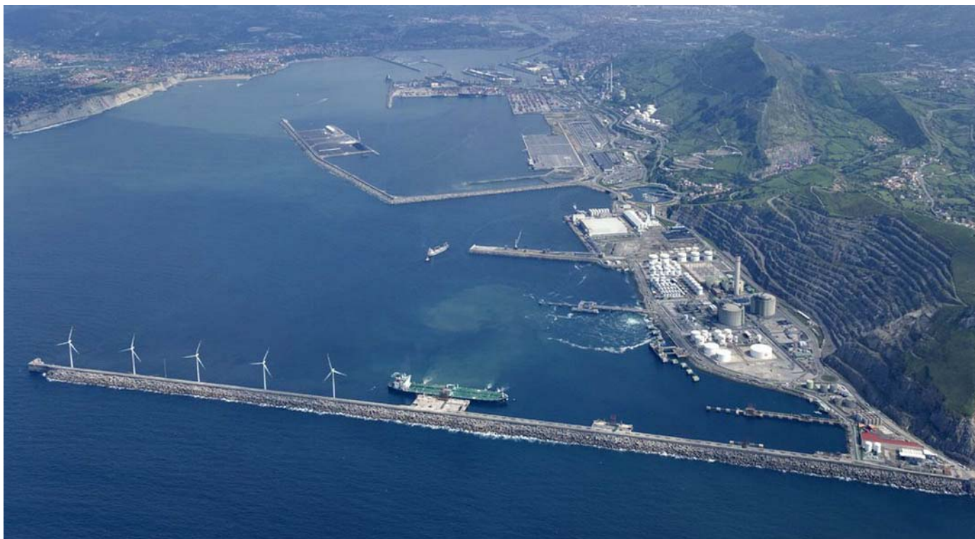
Bilbao—Punta Lucero Breakwater from W
