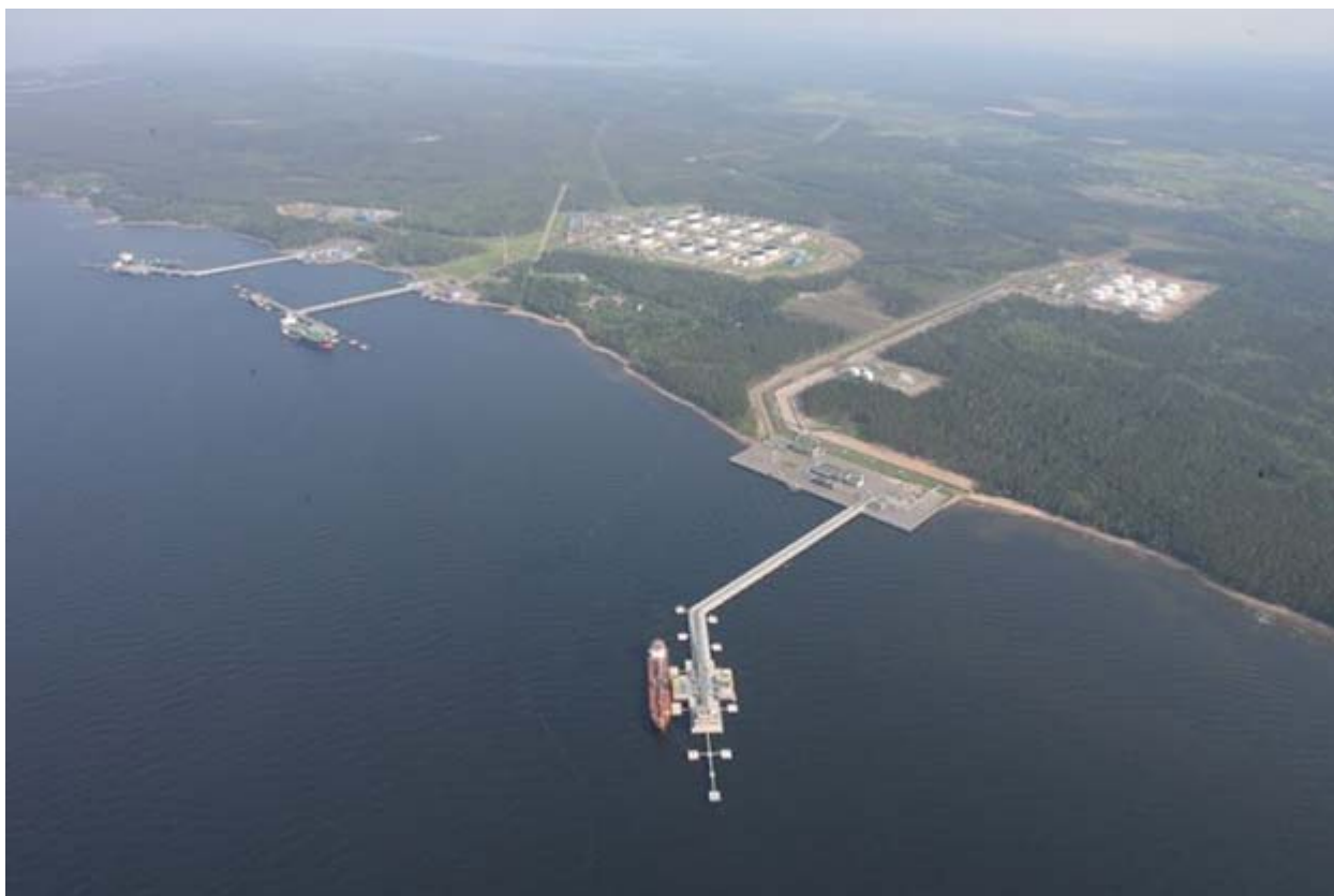
Primorsk Oil Terminal
