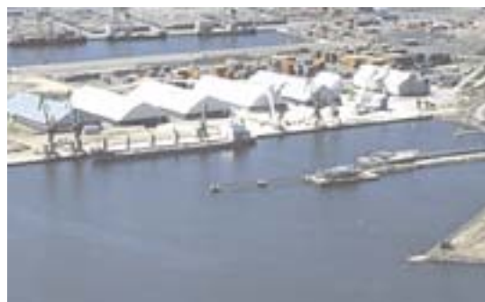
Kotka—Mussalo (dry bulk terminal)
