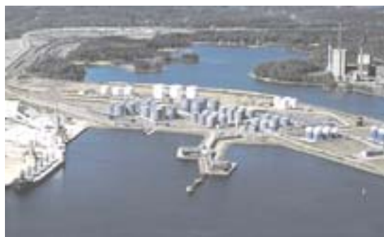
Kotka—Mussalo (oil terminal)
