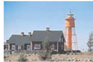
Rodkallen Disused Light Tower
