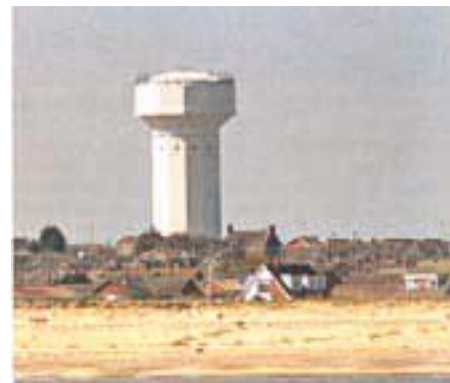
Caister water tower
