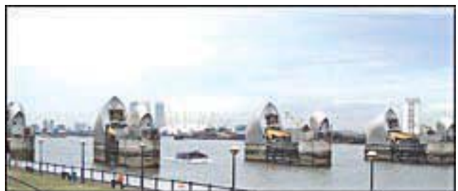
Thames Tidal Barrier
