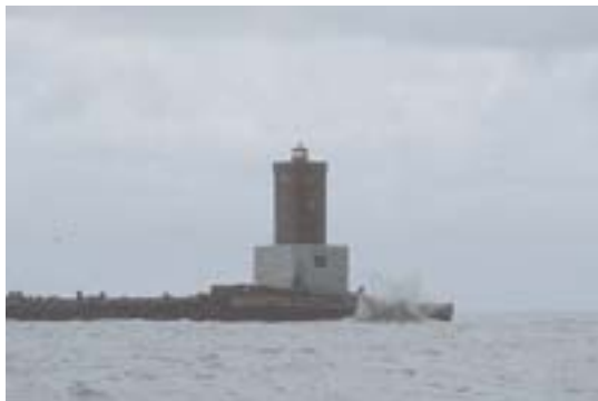
Minsener Oog Disused Light Tower (Buhne A)
