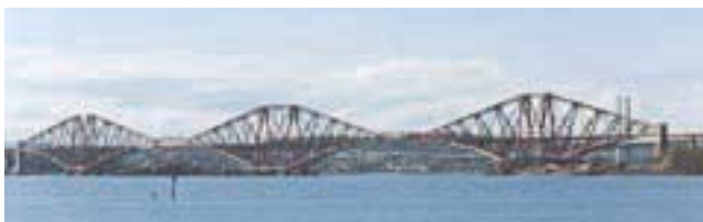
The Forth Bridges from NE
