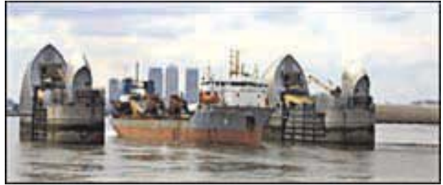
Thames Tidal Barrier (passage open)
