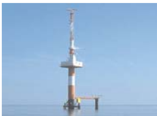
Hookseilplate Radar Tower
