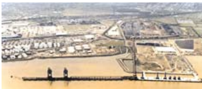
Immingham Bulk Terminal
