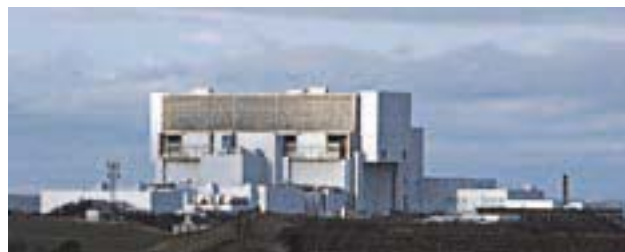
Torness Nuclear Power Station
