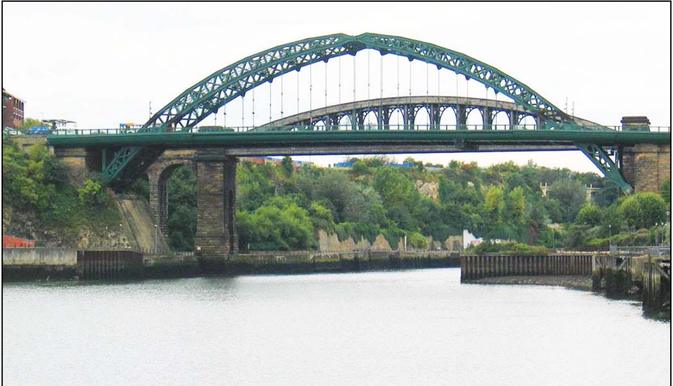
Sunderland Railway Bridge
