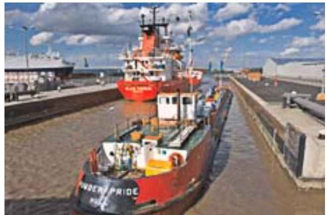
Hull—King George Dock Lock (HW)
