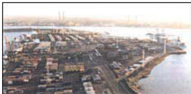
Northfleet Hope Container Terminal
