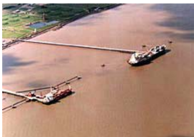
South Killingholme Oil Terminal
