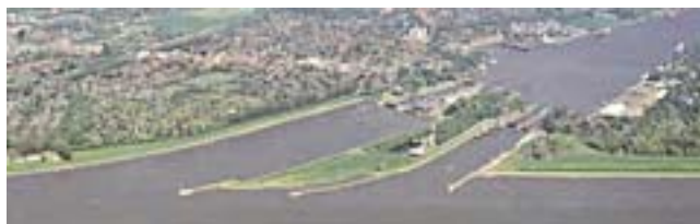
Canal entrance at Brunstüttel
