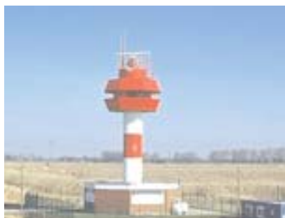
Wybelsum Radar Tower (Emden)
