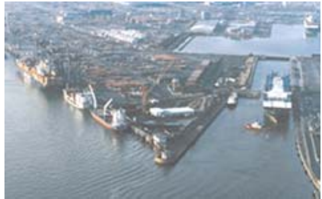
Bremerhaven—Nordschleuse (North Lock)
