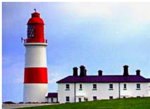
Souter Disused Lighthouse (Lizard Point)
