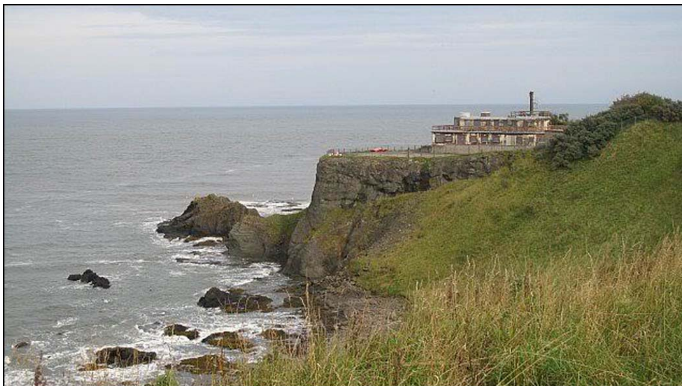
Ginhead—Stack and Buildings
