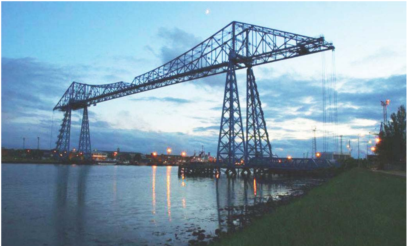
Tees Transporter Bridge
