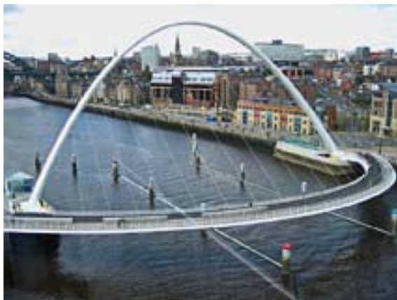
Gateshead Millennium Bridge (closed)
