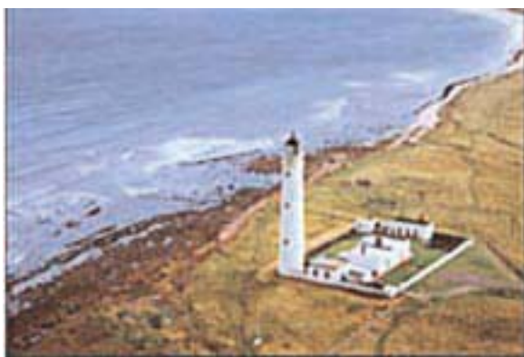
Barns Ness Disused Light Tower
