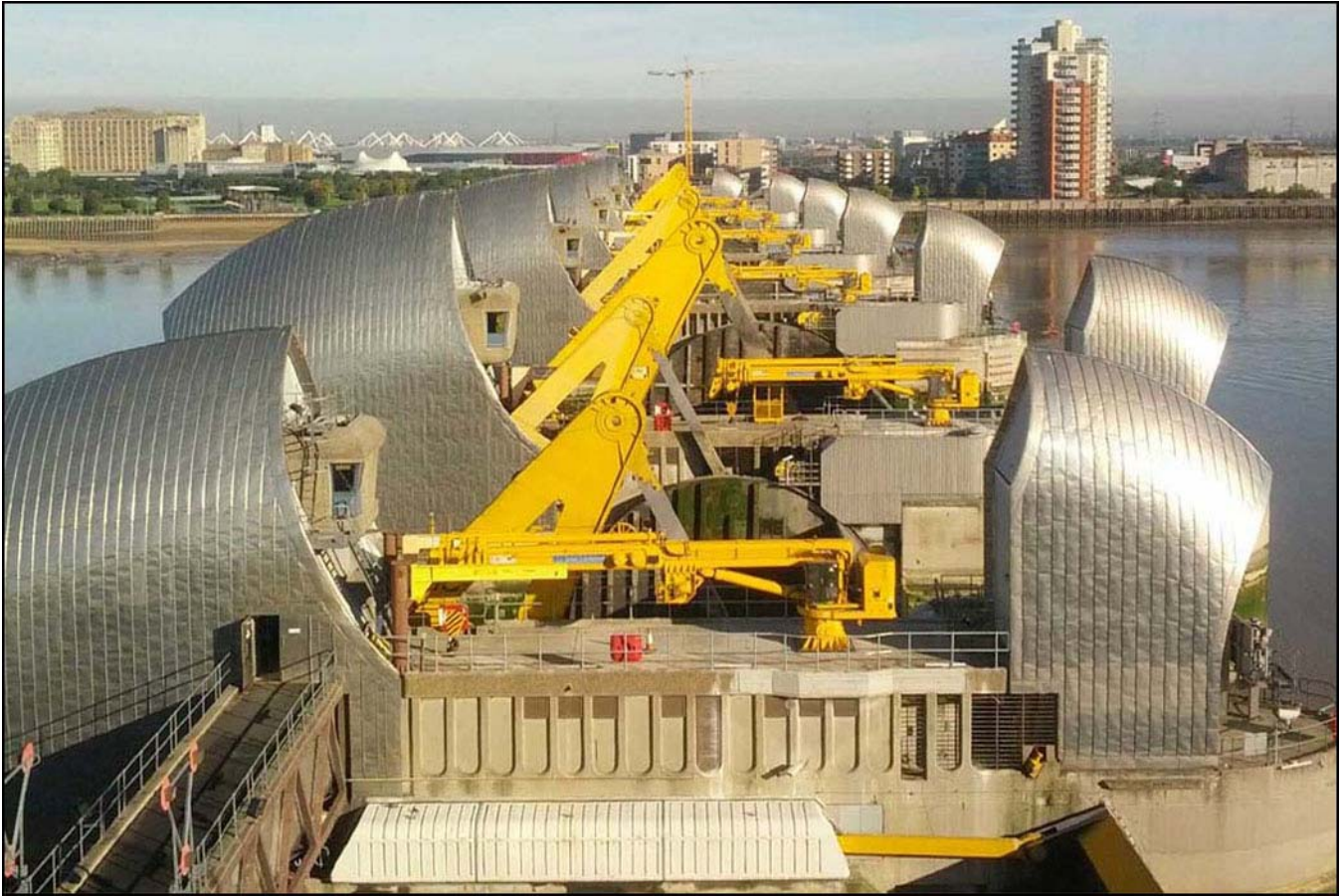
Thames Tidal Barrier from E
