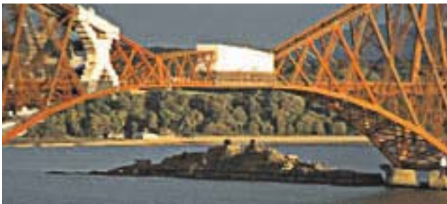
Inch Garvie (under the Forth Railway Bridge)
