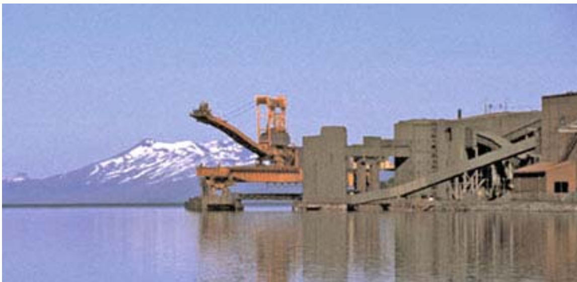
Narvik—Iron Ore Terminal
