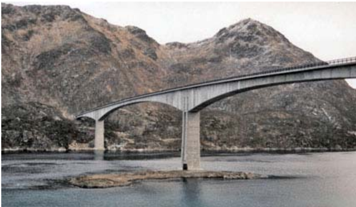
The Raftsundet Bridge from S
