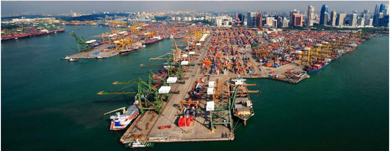
Tanjong Pagar— Container Terminal
