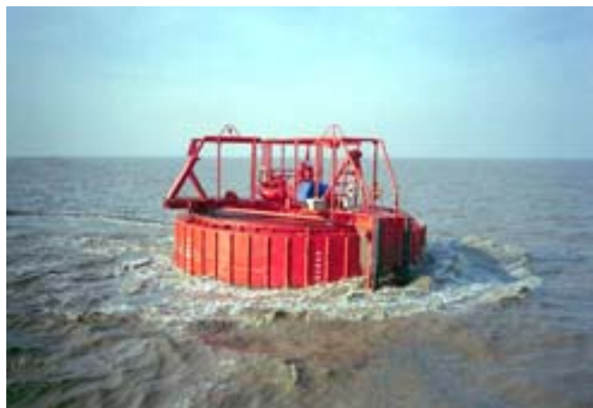
Hazira Offshore Terminal SPM
