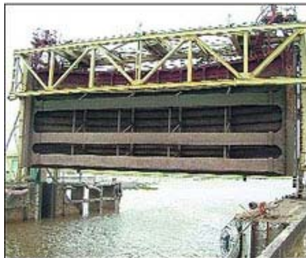
Lock Gate at Bhavnagar Port
