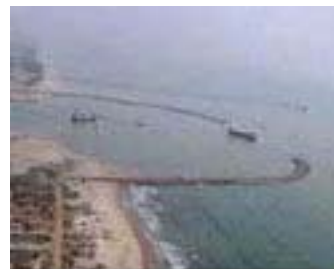
Karaikal Port Breakwaters
