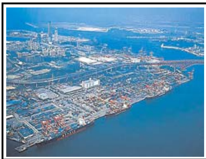
Osaka Ko—East Container Terminal
