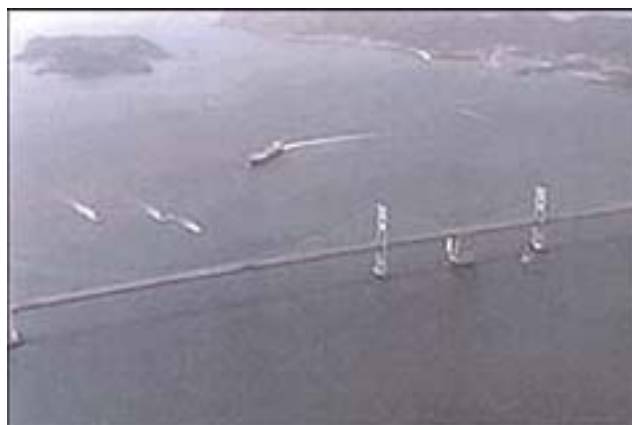
Seto Ohashi Bridge
