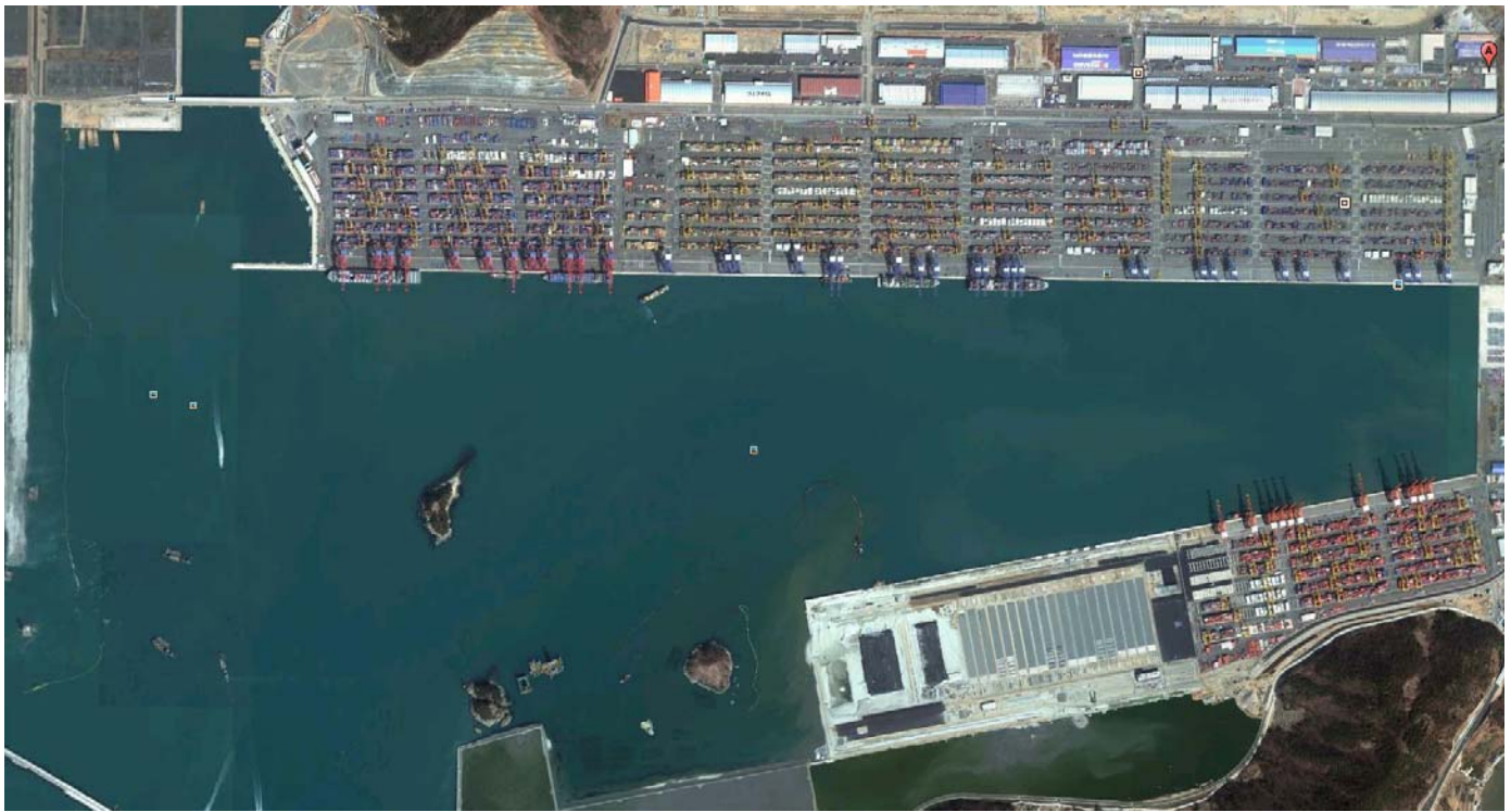
Pusan New Port—Container Terminal
