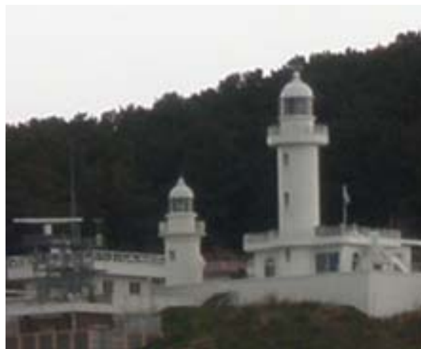
Cheju Hang Traffic Control Center
