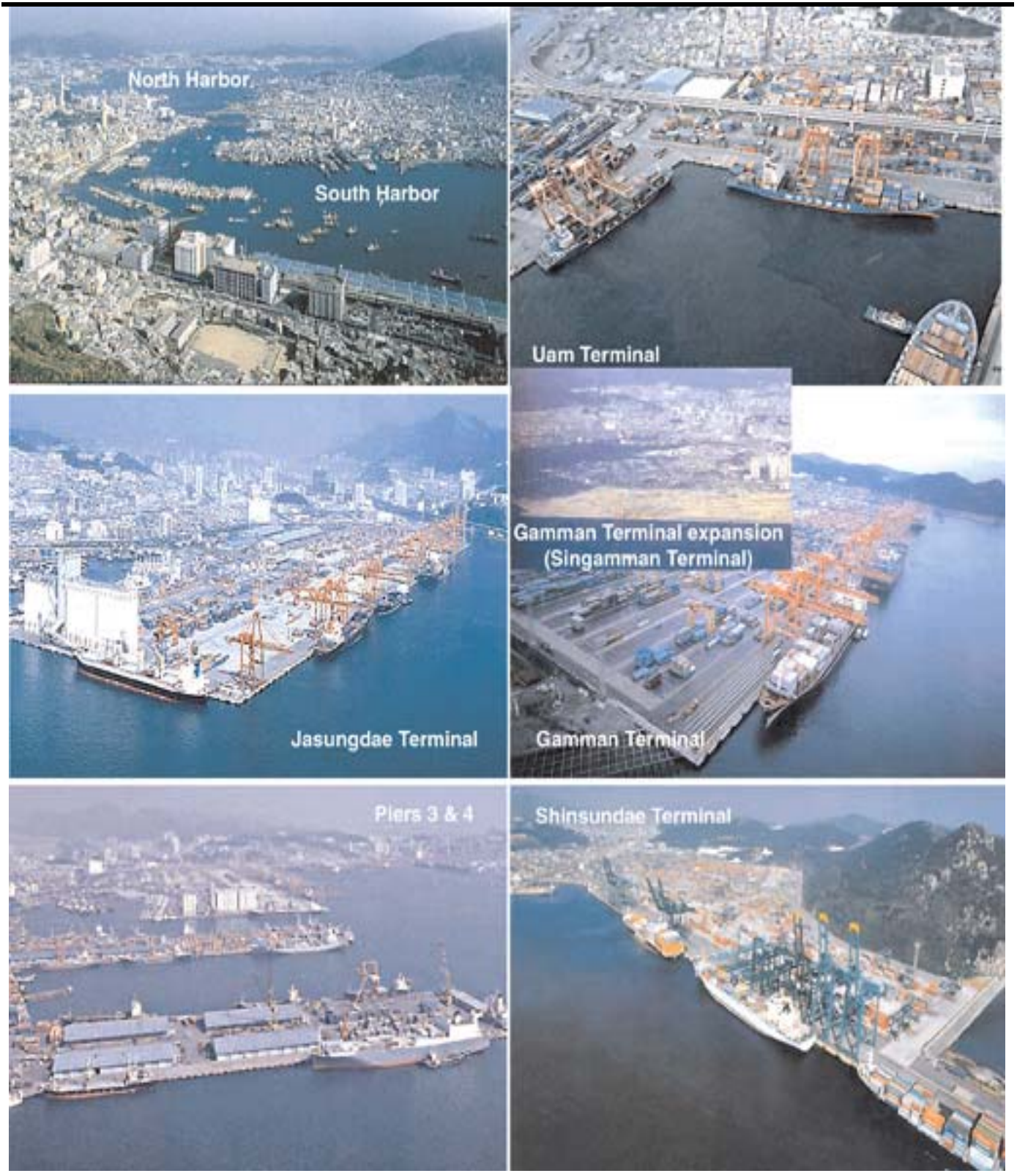
Pusan—North Harbor Terminals
