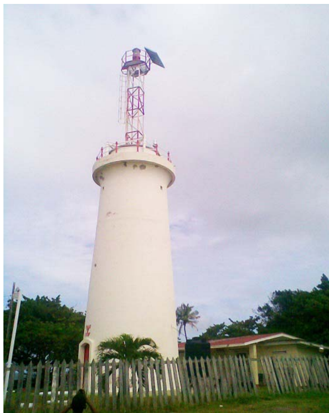
Galera Point Light
