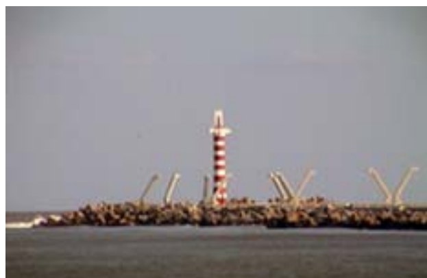
Coatzacoalcos Entrance Light on the breakwater
