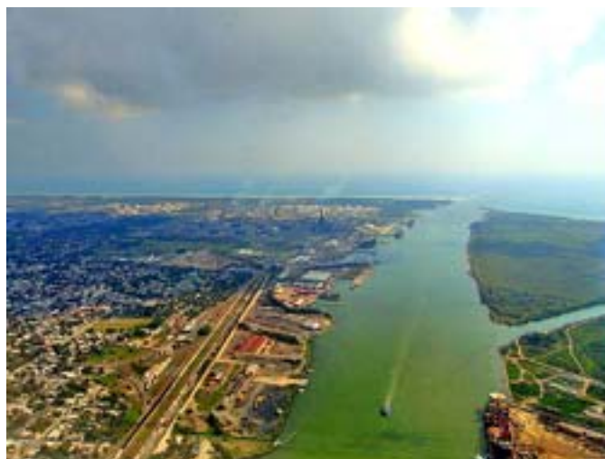
Tampico—from W to E toward breakwater
