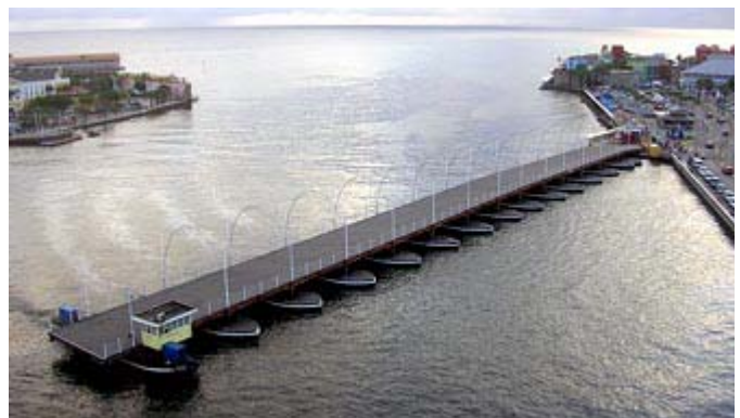
Queen Emma pontoon bridge
