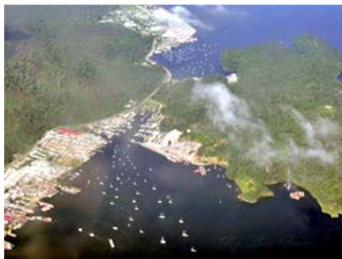
Chaguaramas Terminal Wharf (center)
