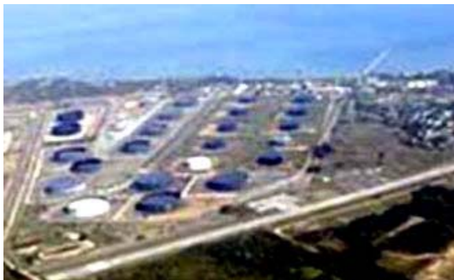
Covenas Tank Farm
