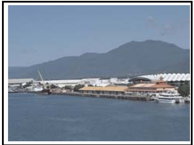
Courtesy of the USS GERMANTOWN Cairns—Berth 1 to Berth 6
