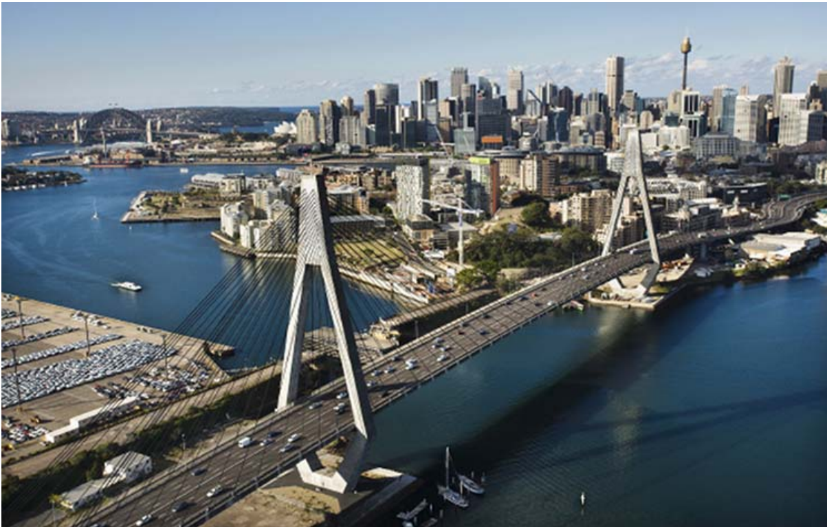
The Glebe Island Bridge from SW
