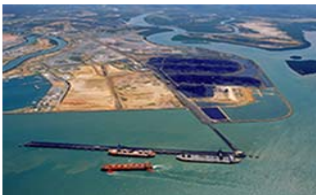
Gladstone—RG Tanna Coal Loading Wharf
