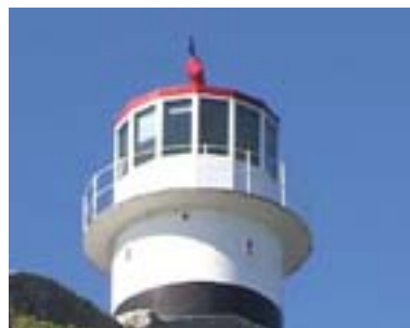
Cape Point Disused Light Structure
