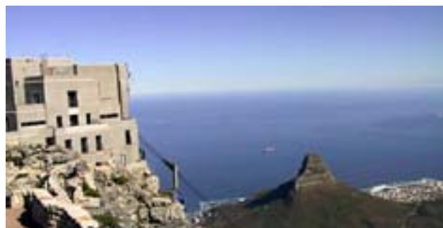
Upper Cable Station (Table Mountain)
