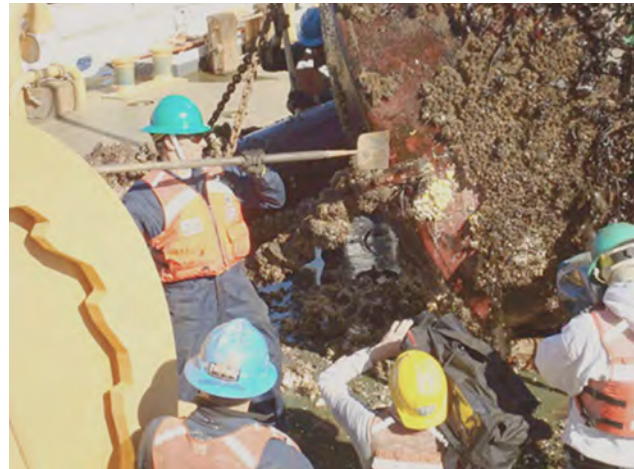
Figure 809. USCG removing marine growth from a buoy.
